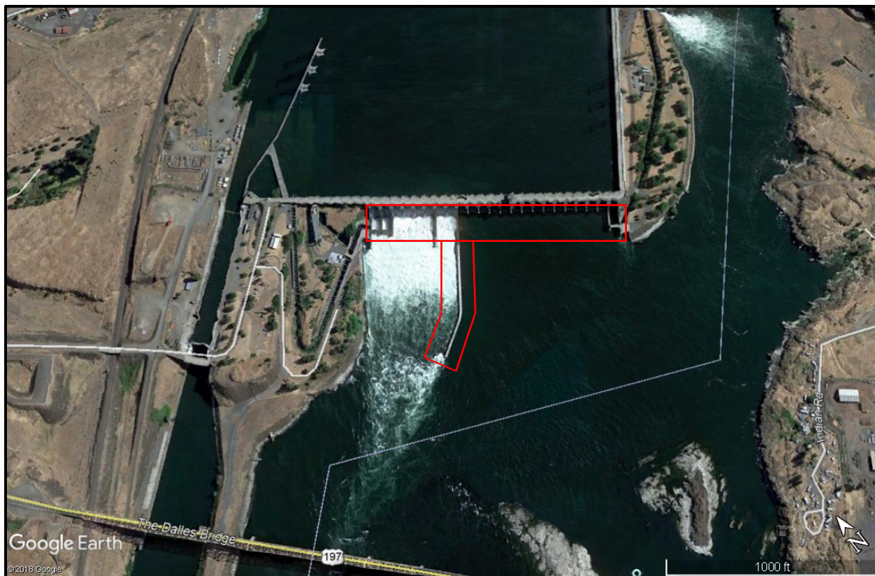
Figure 2 The Dalles Dam Spillway. Red box indicates approximate area of inspection coverage.
